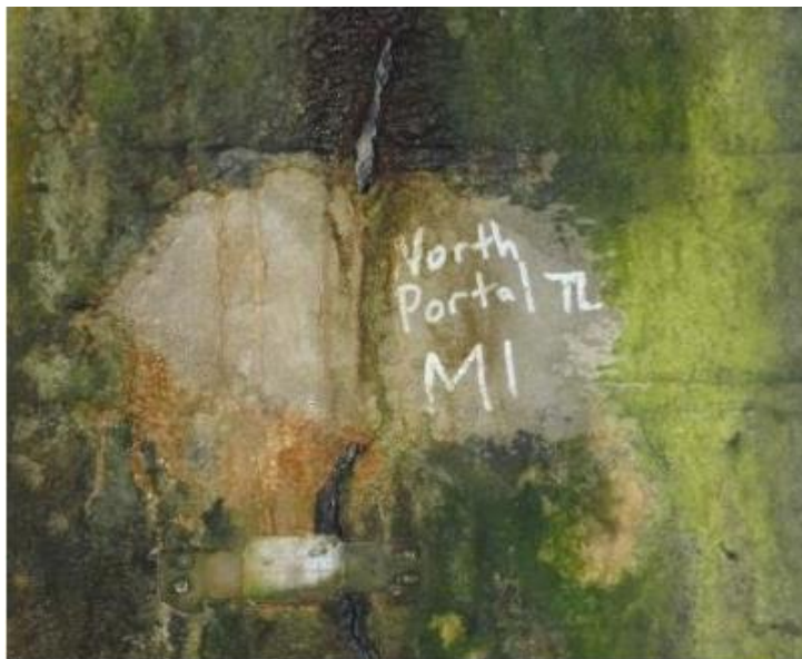
Picture 10: North Portal mortar crack pad monitoring crack lengthening
