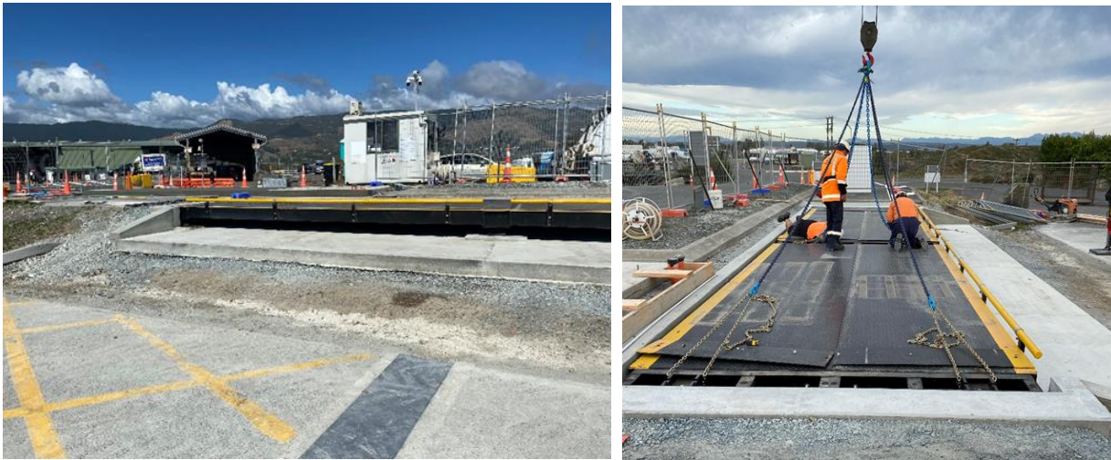
Figures 5 and 6: Richmond RRC weighbridge showing concrete base with crossfall for easy maintenance (left), lifting weighbridge into place (right)
