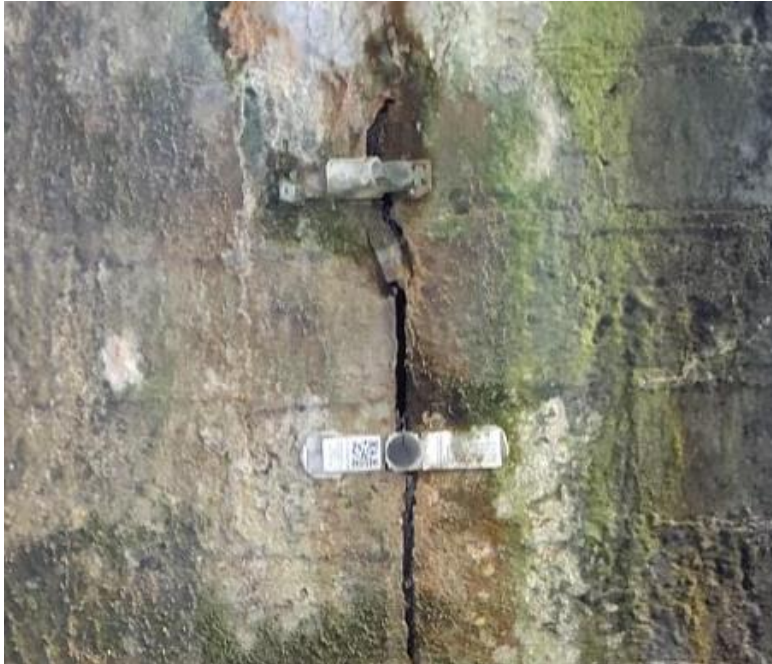
Figure 11: Typical Moire tell-tale monitoring crack width
