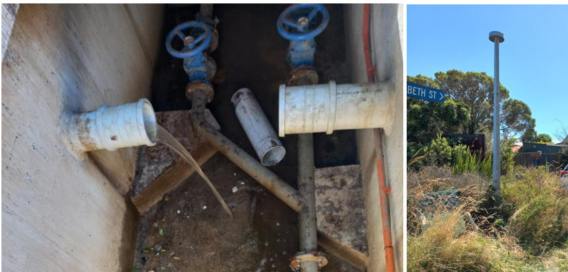
Figure 1 (left): water infiltration into pump station. Figure 2 (right): the source of water infiltration.
