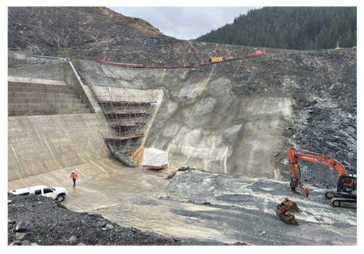
Figure 9: Plunge pool works being completed, October 2023
