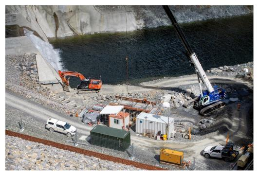
Figure 10: Water flowing from the flip bucket into the completed plunge pool, January 2024
