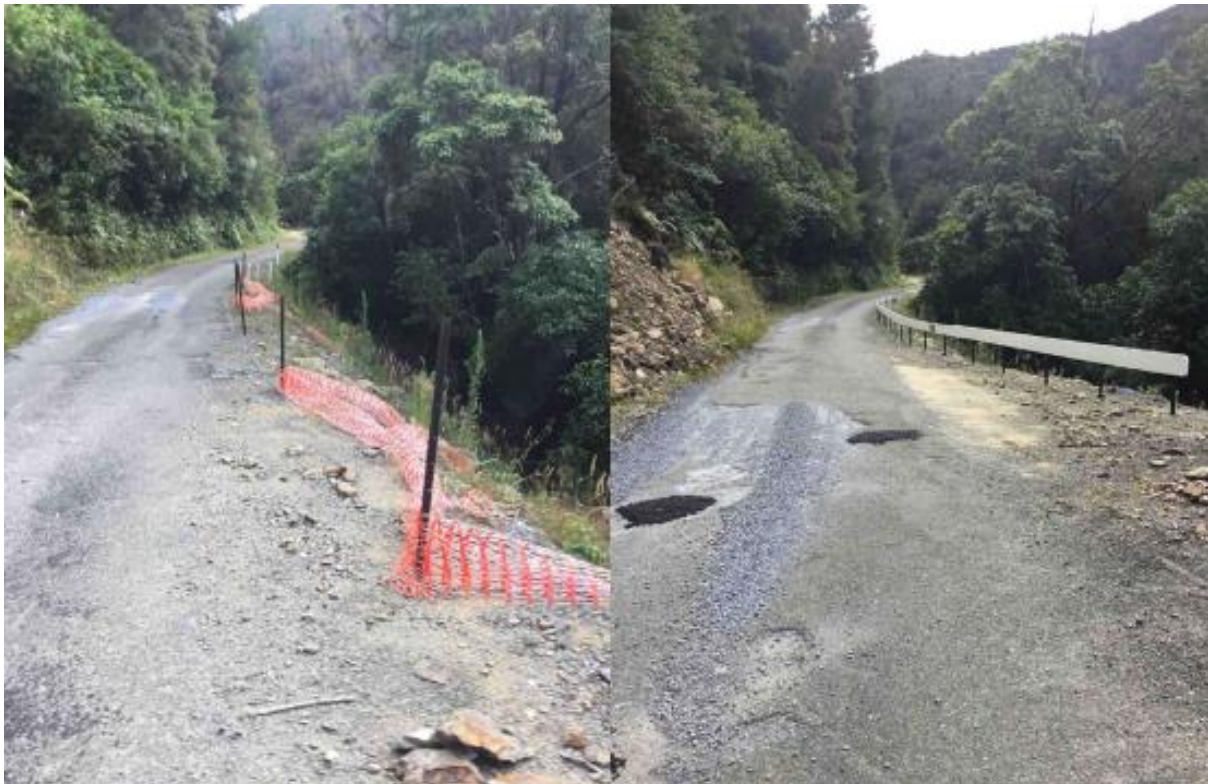
Figure 11 & 12 Cobb Dam Road – broken barrier repair
