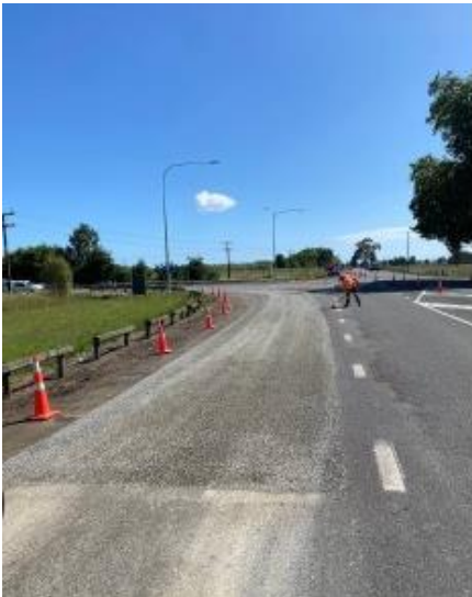
Figure1 – Pre reseal stabilisation repair first coat – Waimea West Road
