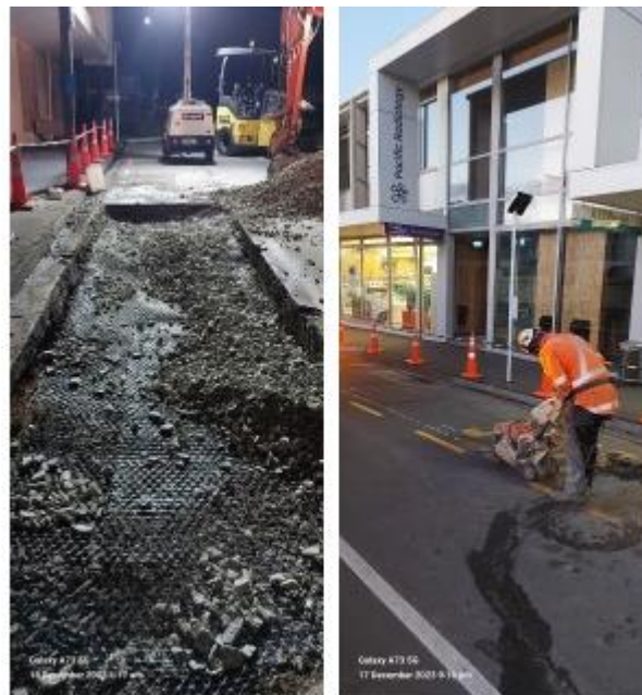
Figure 5 Queen Street Bus Stop dig-out repair – December 2023
