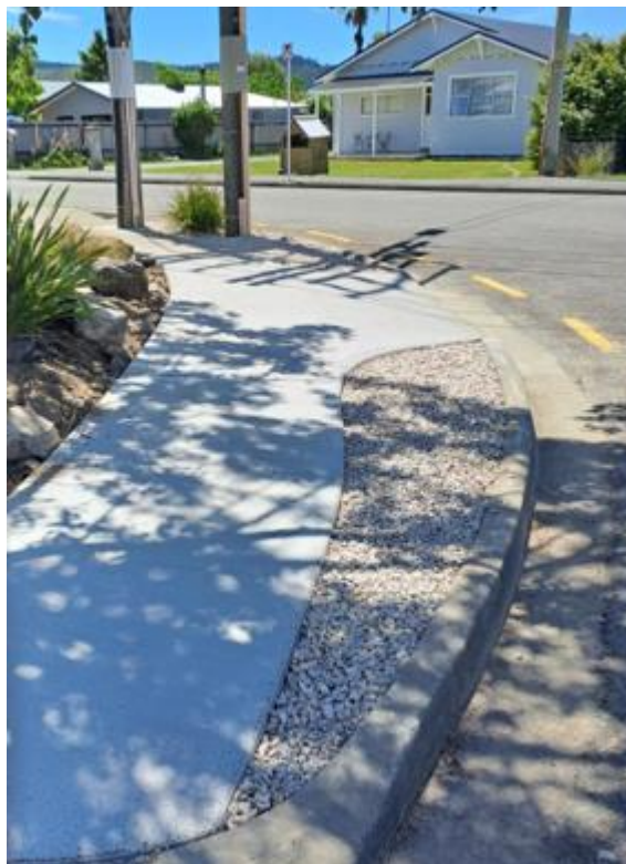
Figure 6 Newly installed pram ramp
