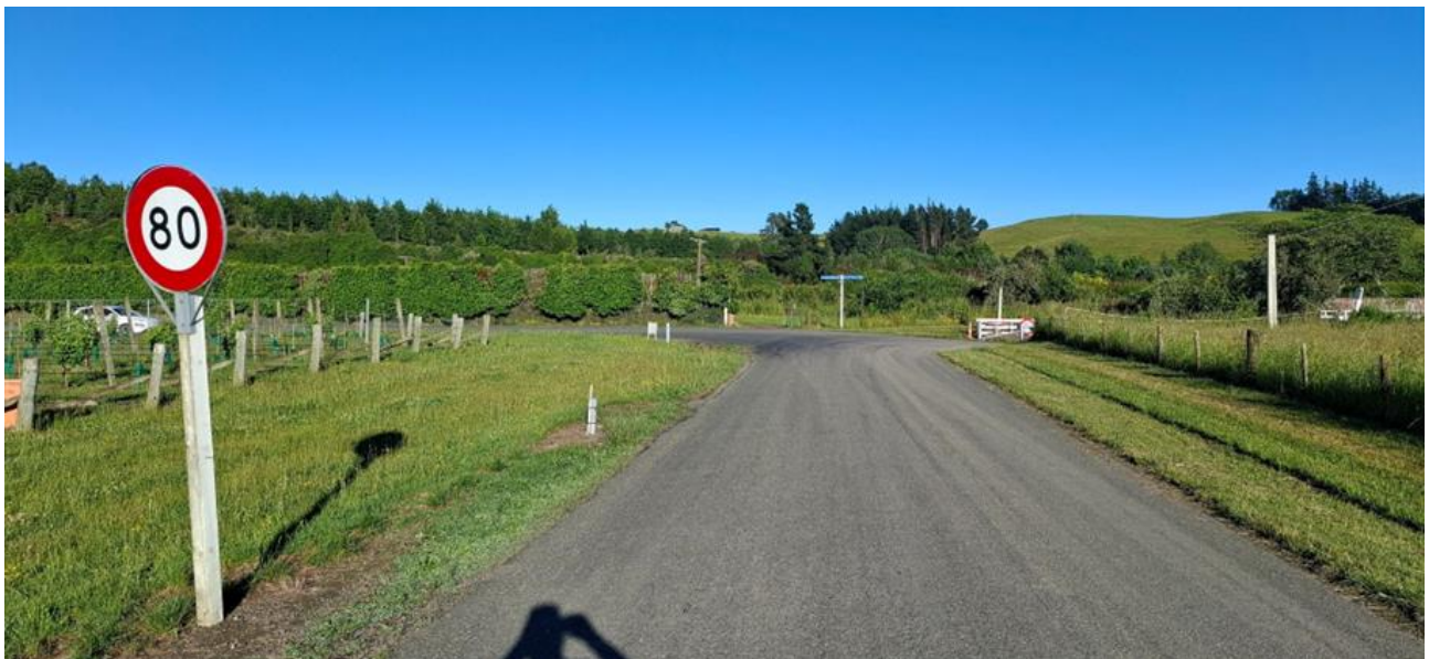
Figure 19: View along Challies Road to its intersection with Golden Hills Road
