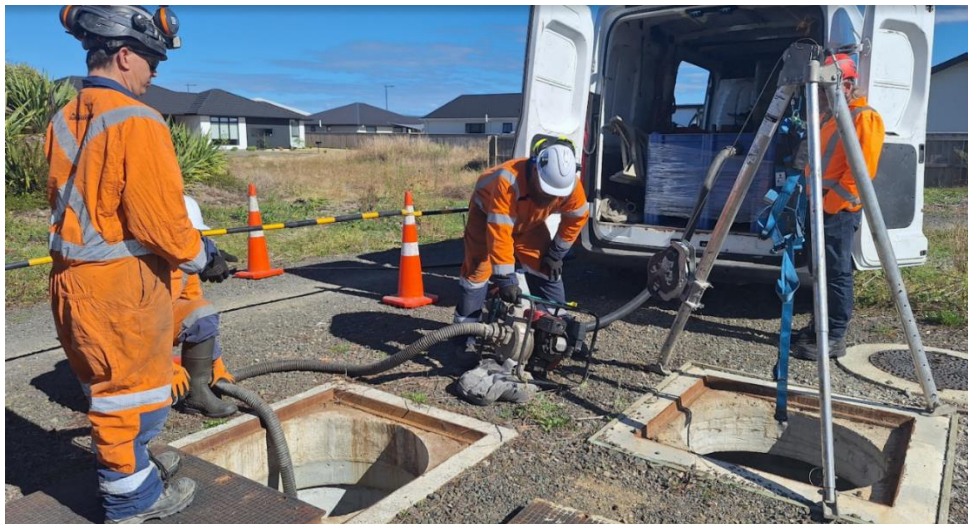
Figure 5: Contractor’s cleaning out the stormwater treatment devices (Jellyfish and Cascade Separator)
