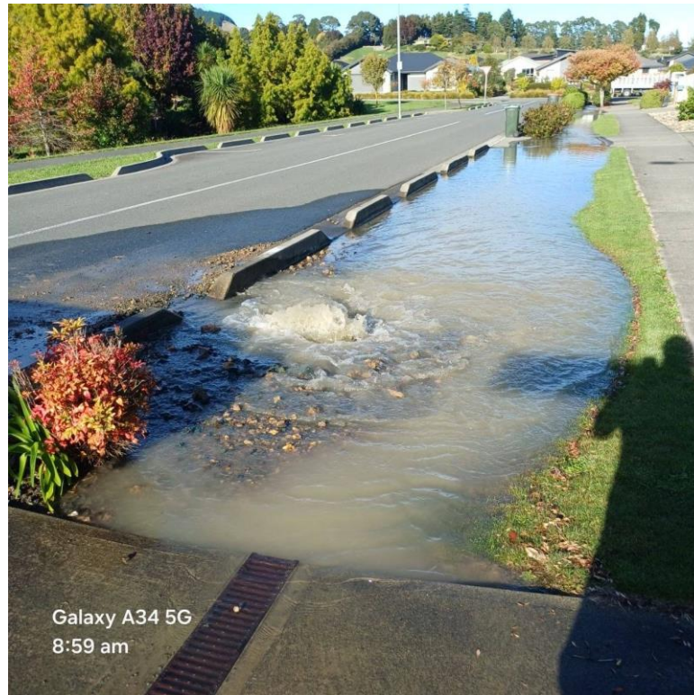
Figure 1: Burst outside 5 Fairose Drive
