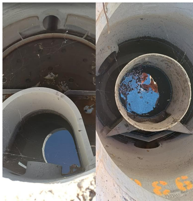
Figures 6 (left): Jellyfish membrane filter. Figure 7 (right) Cascade separator
