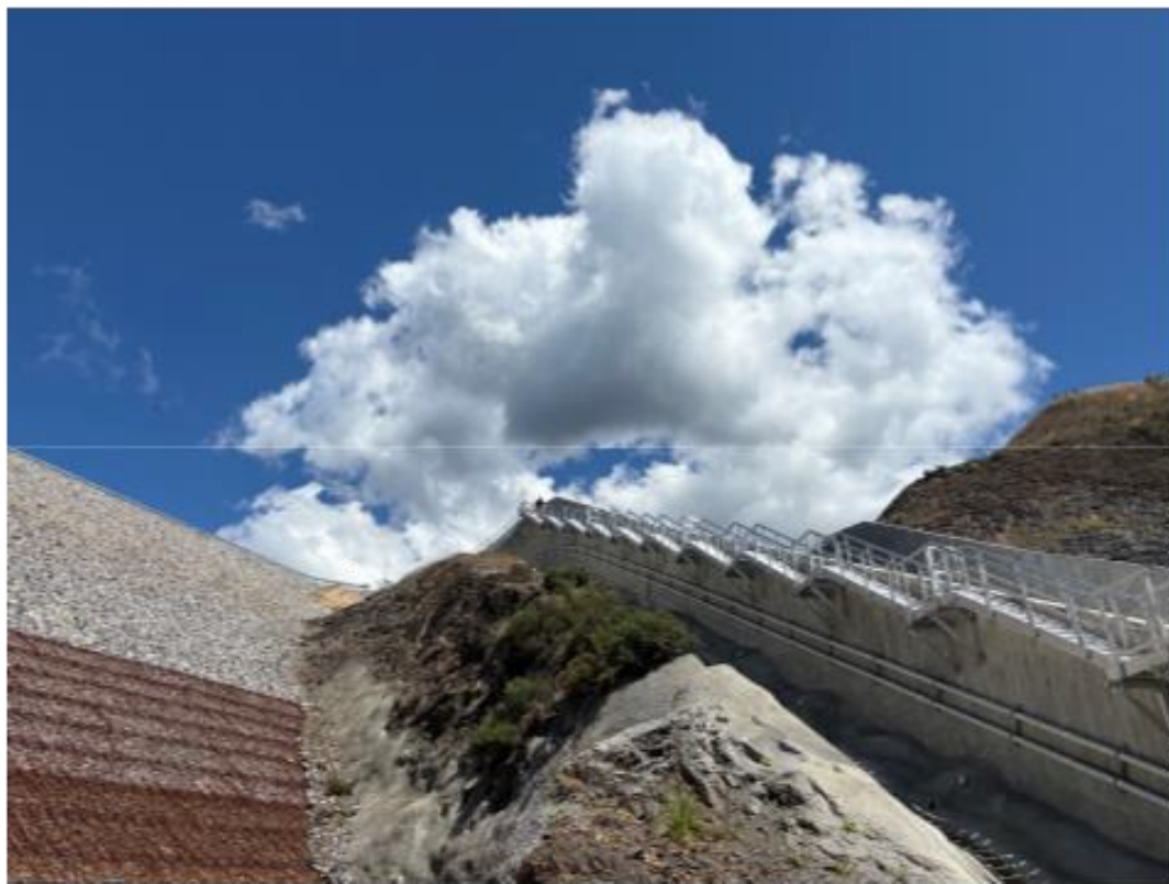
Figure 1 Looking up at the spillway stairs
