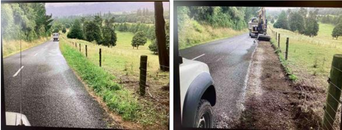
East Takaka flanking to improve drainage
