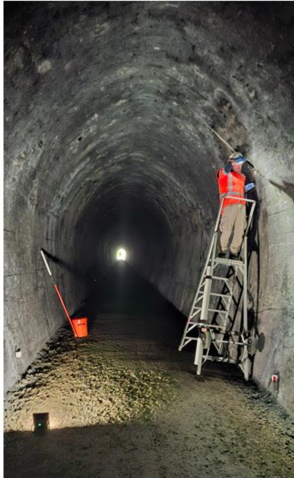
Regular tunnel measurements monitor the tunnel shape
