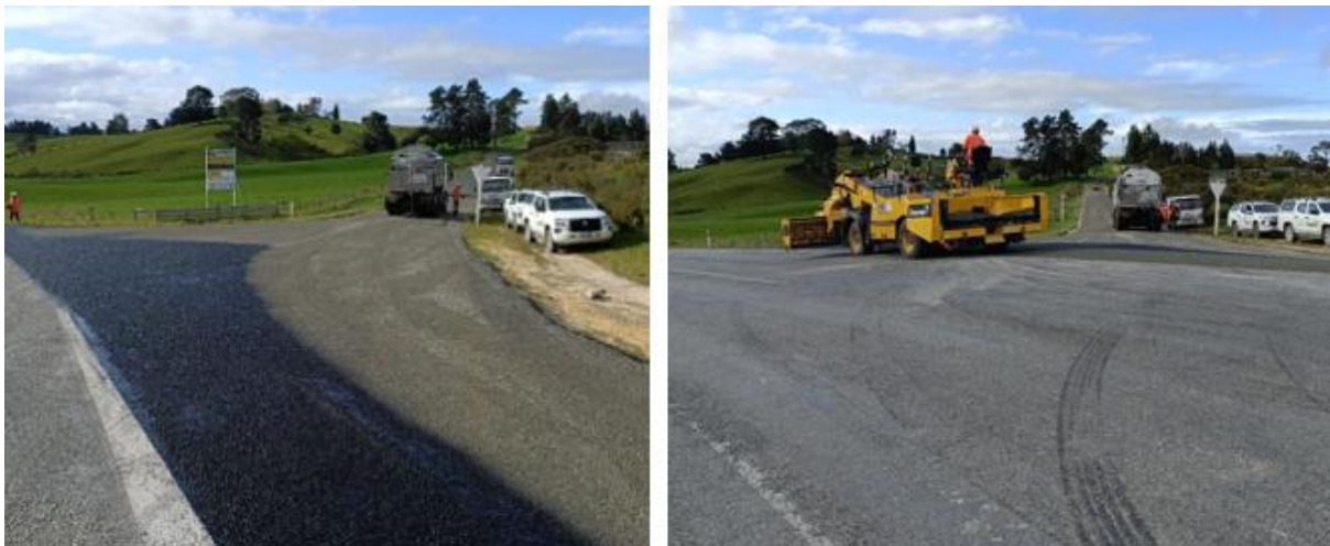
Moutere Highway sealing in progress
