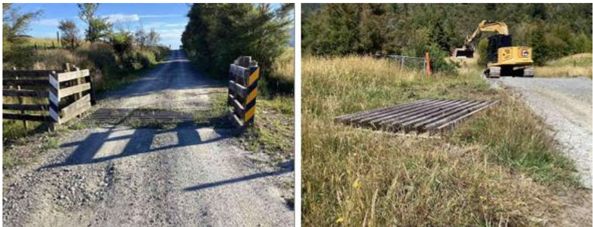
Long plain Road – removal of unused cattle stop
