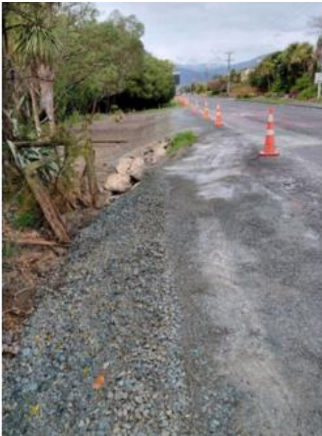
Waimea West Road dropout repair
