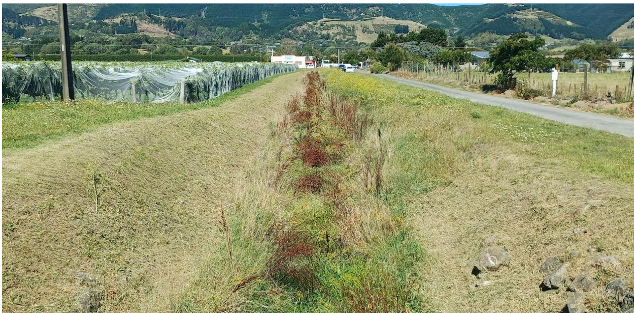
Figure 3: Example of a good balance of open channel maintenance
