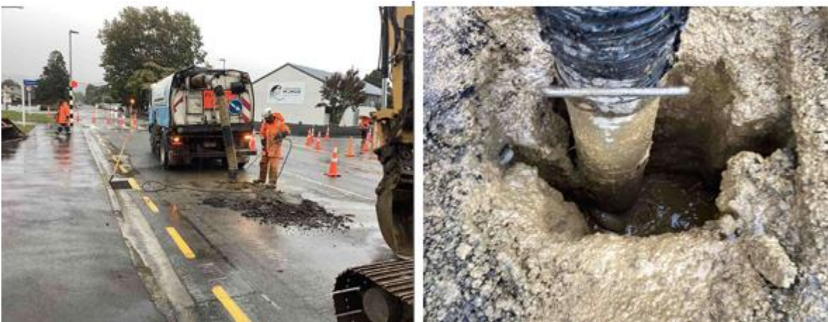
Meihana Street test pits
