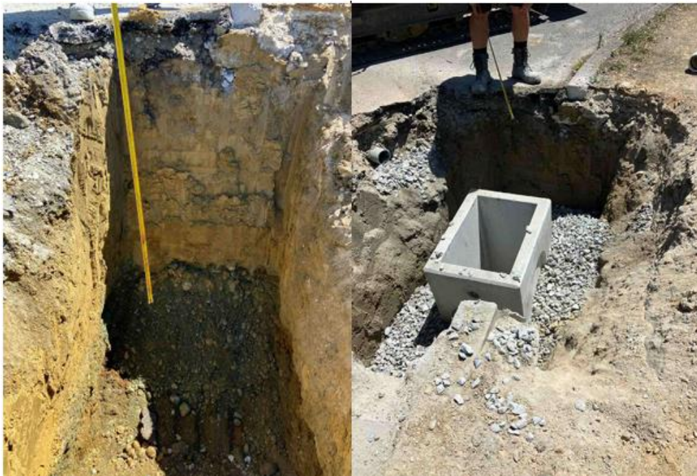
Meihana Street/Rototai Road intersection – new sump
