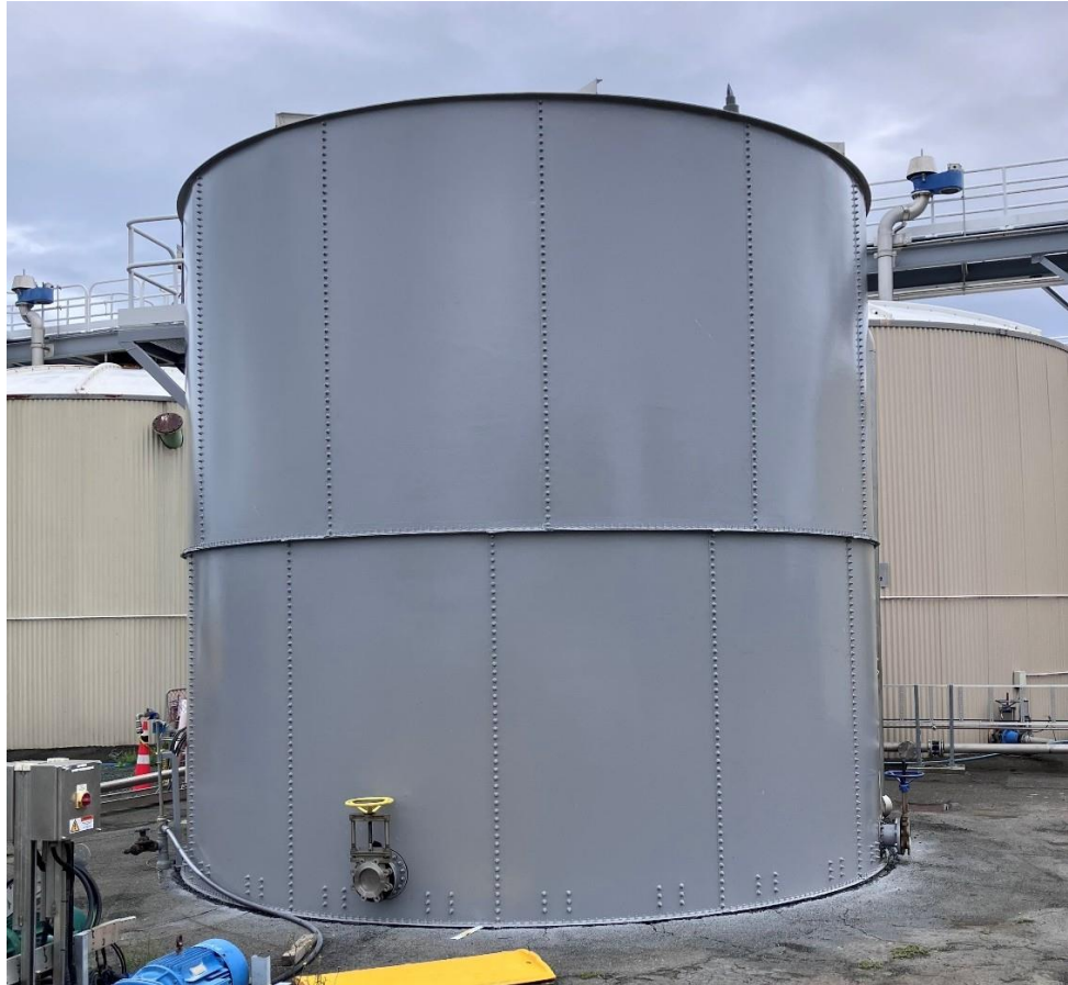
Figure 3: Refurbished biosolids tank
