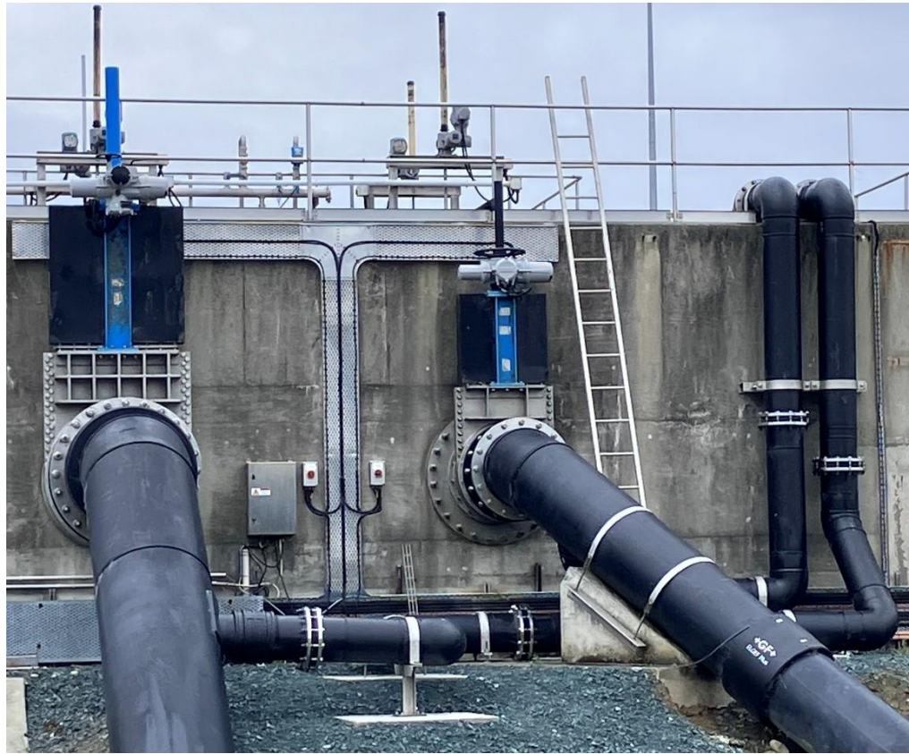
Figure 2: Completed inlet isolation valves and over-pressure protection
