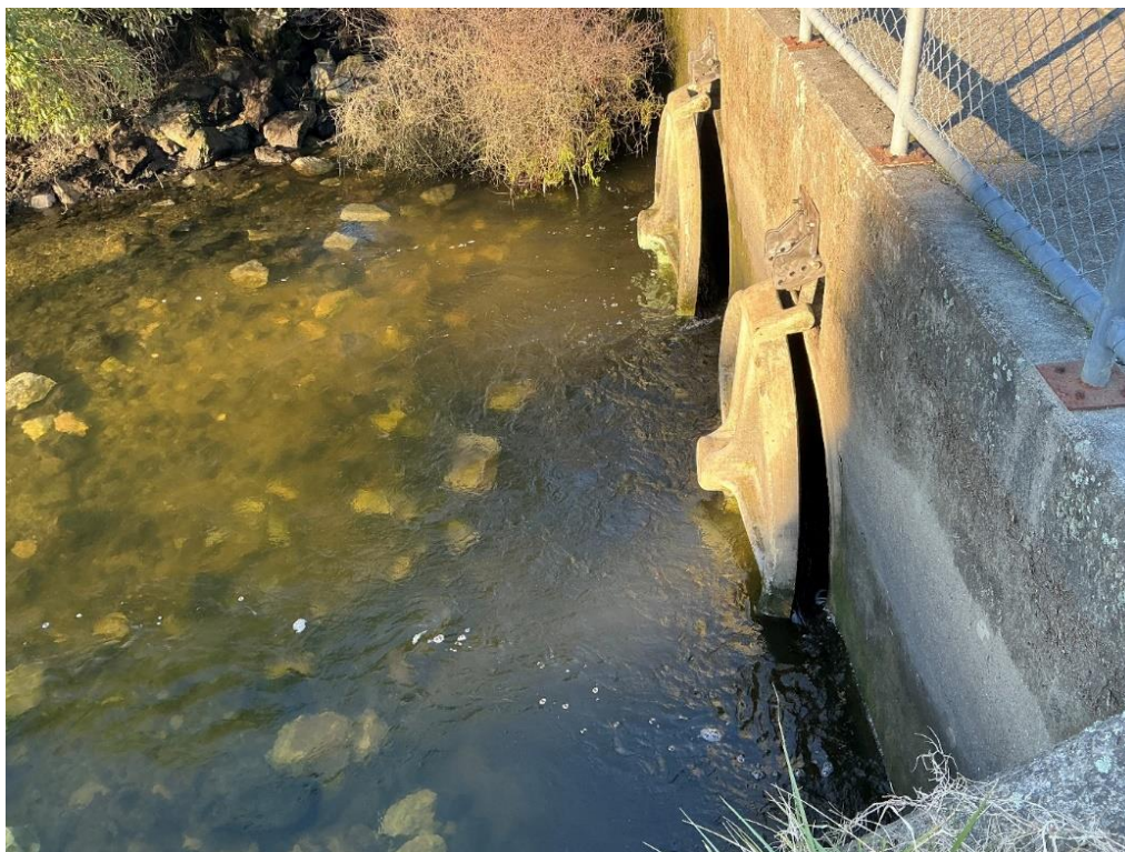
Figure 6: Ferrer Ck tidal gate improved
