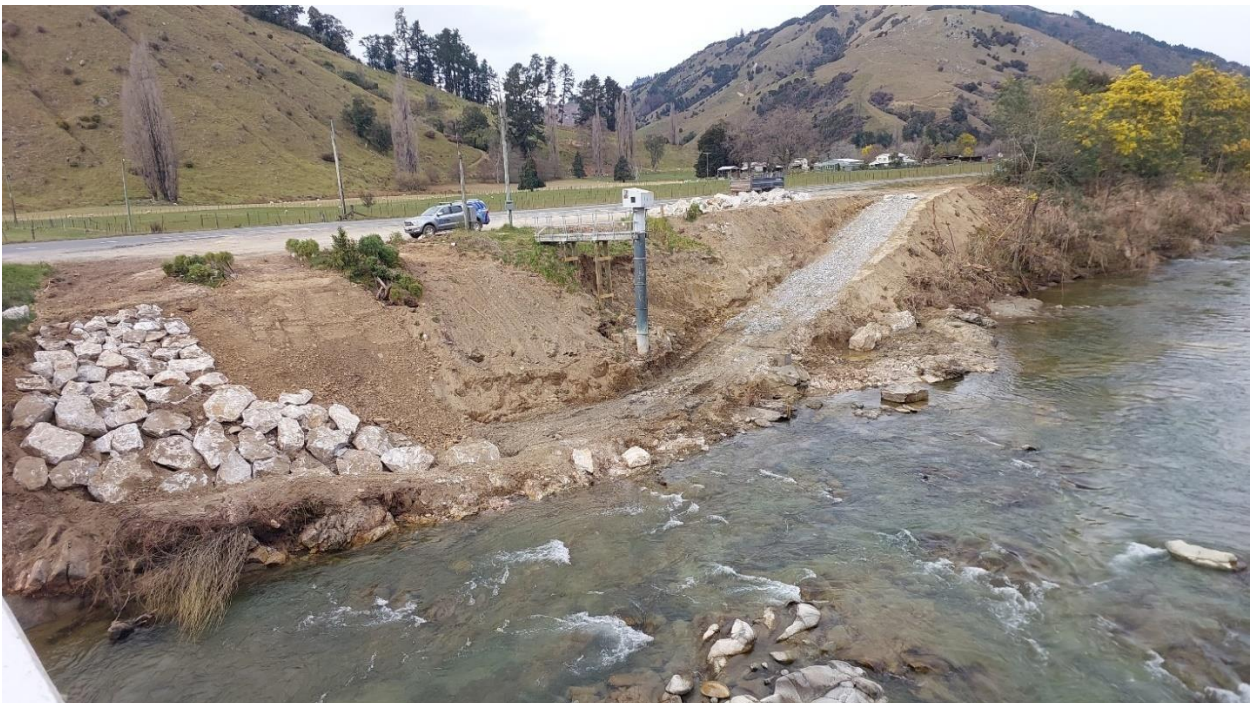
Figure 3: Rock placement underway at the Motueka River at Woodstock flow monitoring station.
