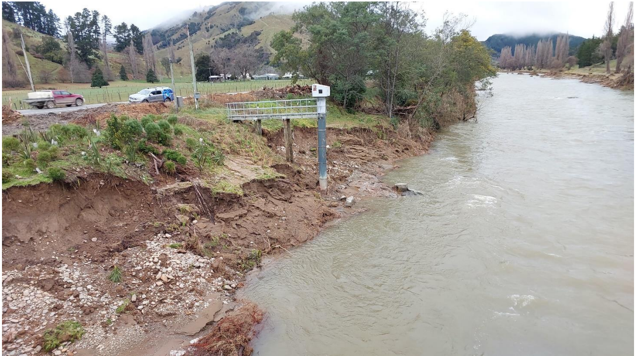
Figure 2: Bank erosion at the Motueka River at Woodstock flow monitoring station after June-July flood events.
