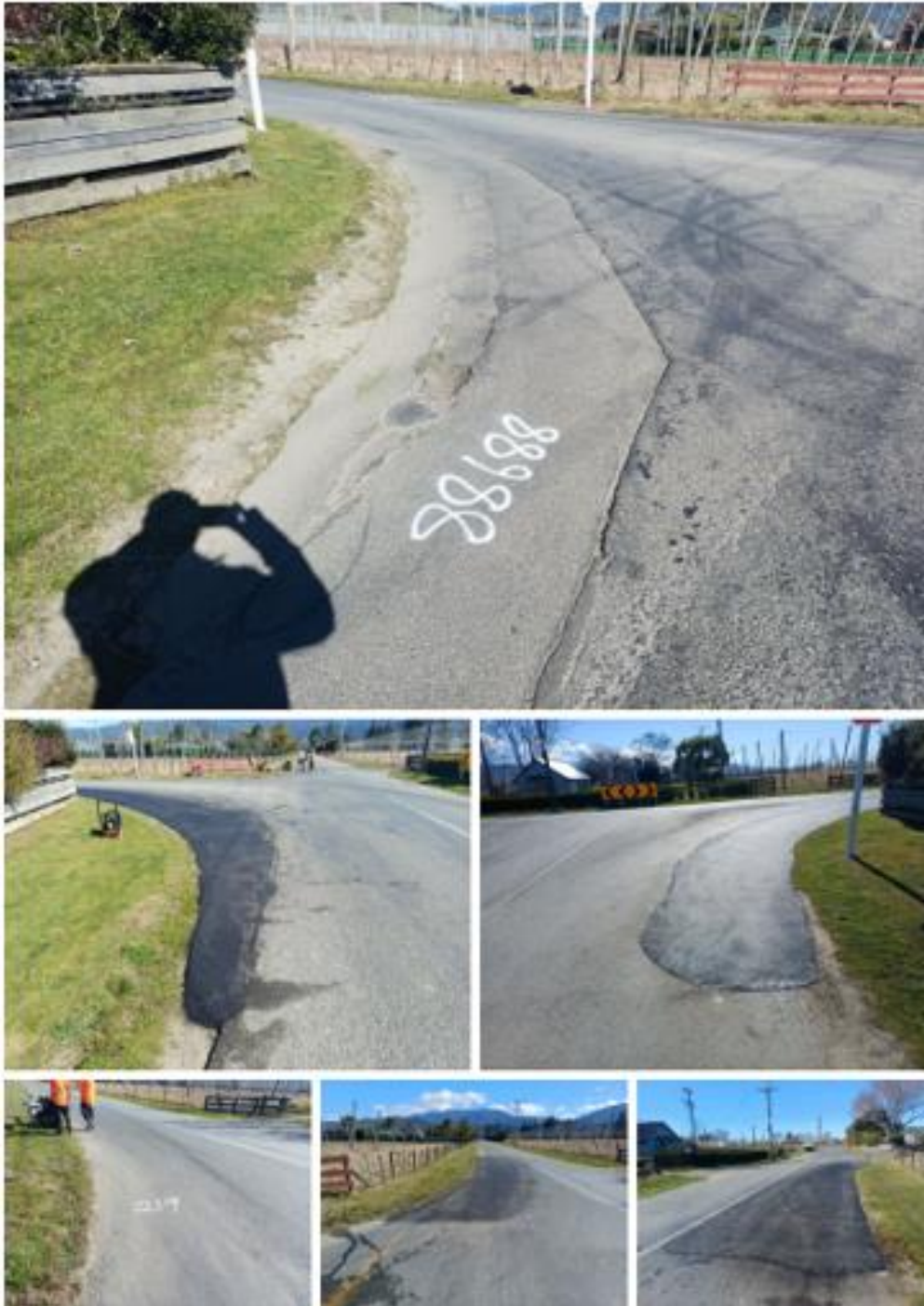
Figure 6: Collection of photos above are all of re-seal repairs on Whakarewa Street
