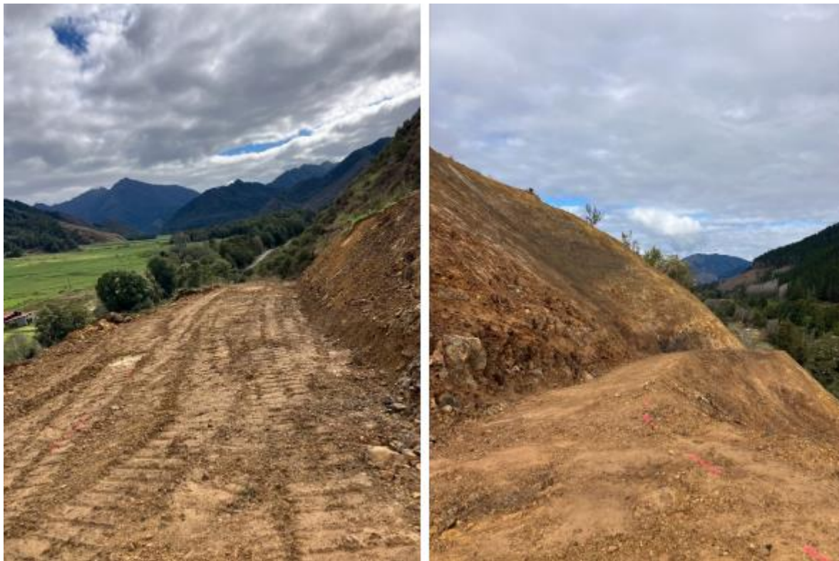
Figure 15: Matiri Valley slip work in progress
