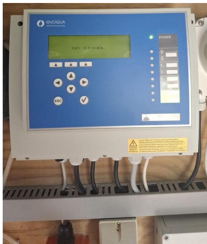
Figure 1: Faulty chlorine instrument "NO SIGNAL"
