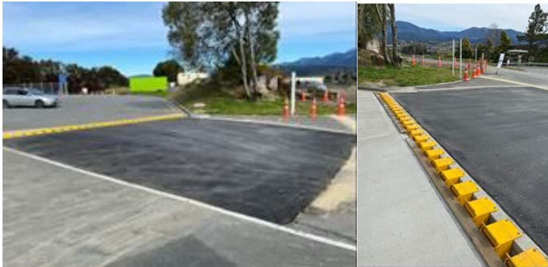
Figures 20 and 21: new traffic control plates at Māiri.
