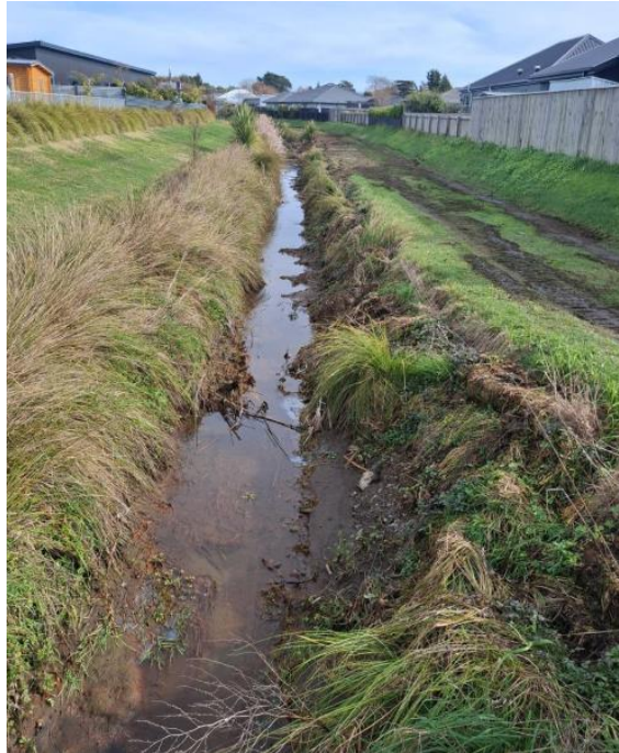
Figure 12: Morley drain, Māpua after clearing
