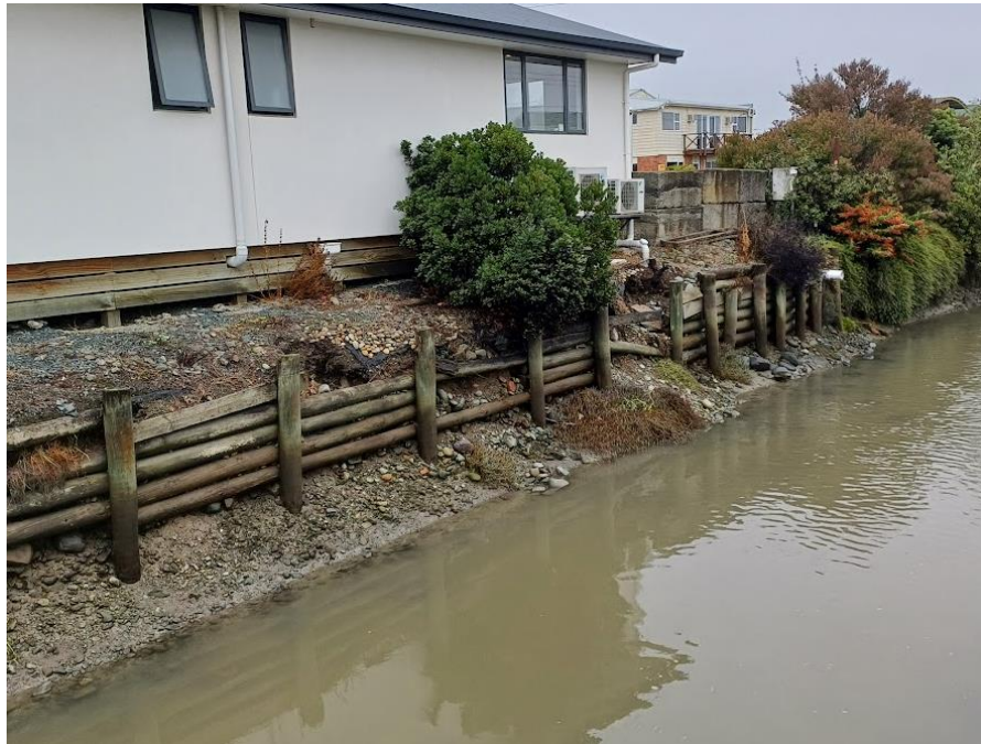
Figure 15: example of damaged retaining wall, Beach Roach, Richmond before
