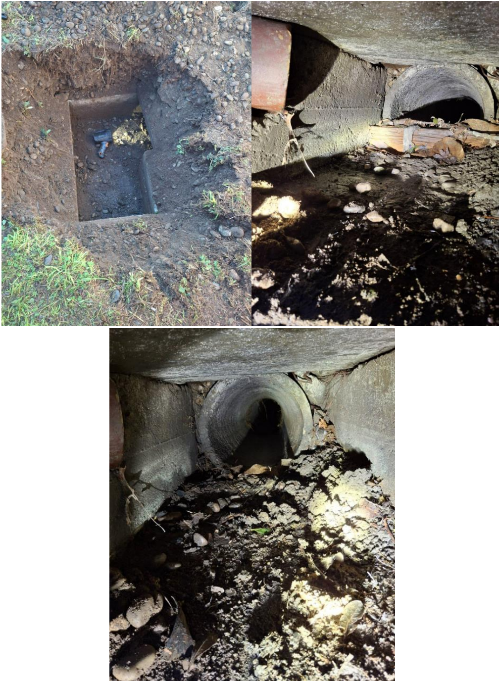
Figures 9 (top left), 10 (Top right) and 11 (bottom): clearing of stormwater at Woodland Avenue
