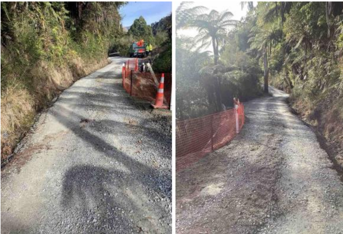
Figure 13: McCallum Road – drop out fenced off
