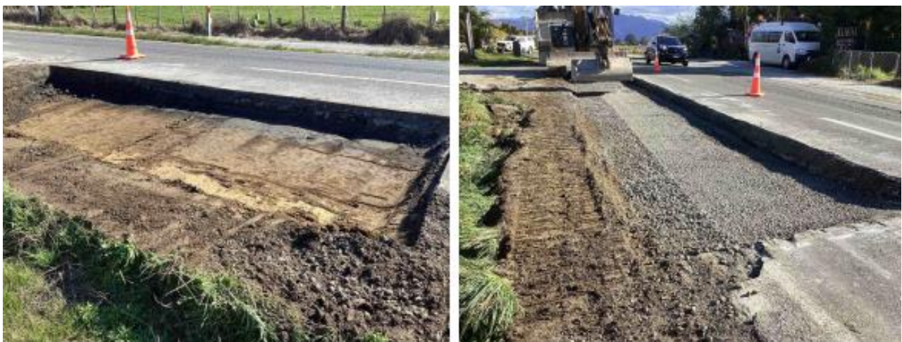
Figure 9: Abel Tasman Drive – pre-reseal repairs
