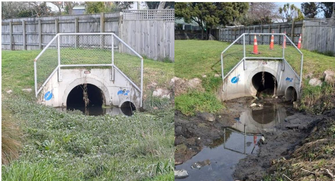
Figures 13 and 14: Morely Drain upstream capacity before (left) and after (right) clearing
