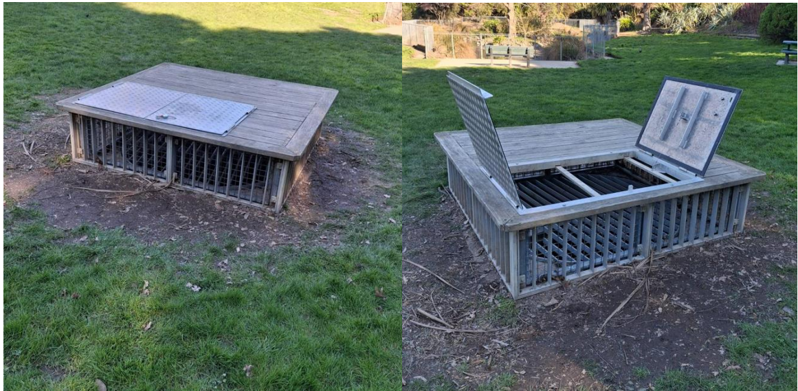
Figures 17 and 18: Washbourn inlet modifications
