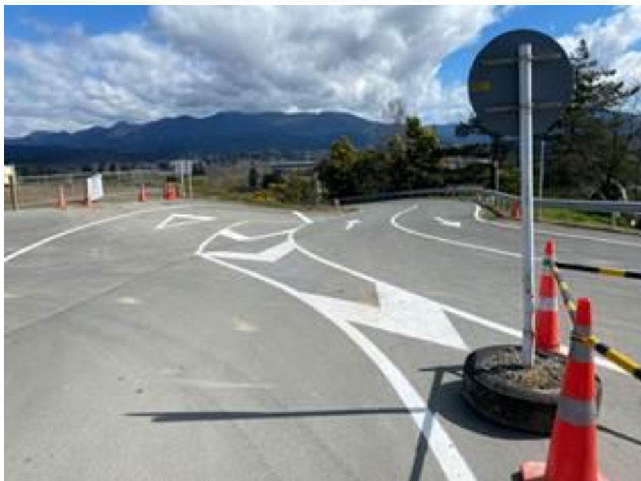
Figure 22: new road markings for the layout
