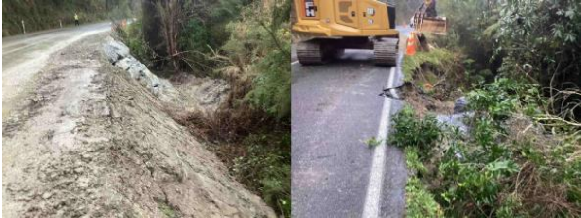
Figure 14: Pupu Valley Road – underslip repairs
