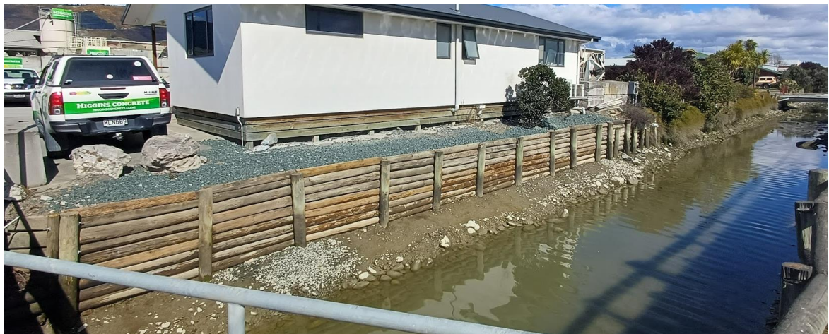
Figure 16: example of repaired retention wall, Beach Roach, Richmond after
