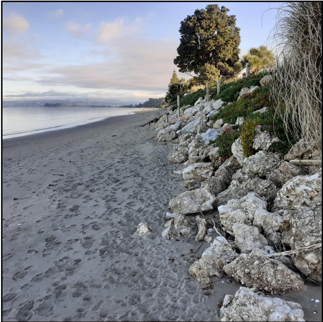
Figure 3: The existing rock protection south of proposed showing the vegetation covering encroaching over the structure to soften the visual impact of the structure. For the proposed rock structure the plants will be coastal indigenous plantings as set out in the landscape planting plan (Appendix 11).
