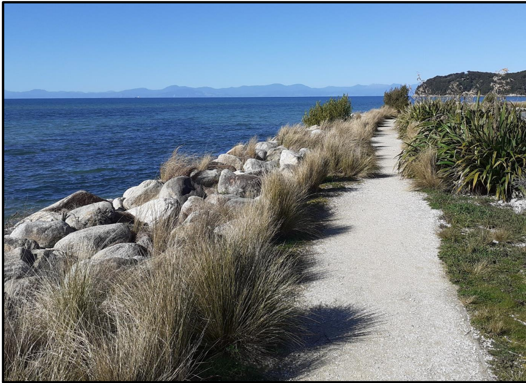
Figure 4: Walkway and coastal planting at the top of the Marahau Rock revetment, which is similar to what will be established on top of the proposed rock revetment.
