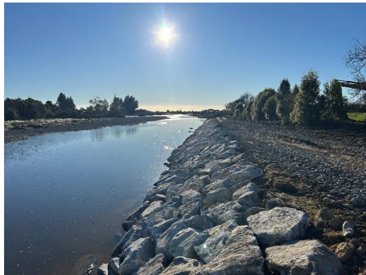
Figures 10 and 11: Erosion at Māriri closed landfill (L) and new rock erosion protection (R)
