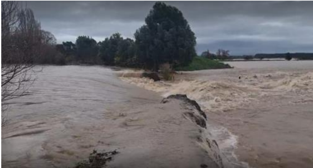
Figure 29: Lower Queen Street to Rabbit Island, water flowing through a gap in the bund that forms the cycle trail
