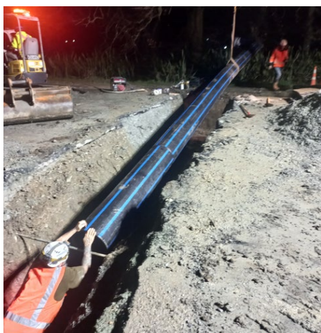
Installation of a raw water main under Lower Queen Street
