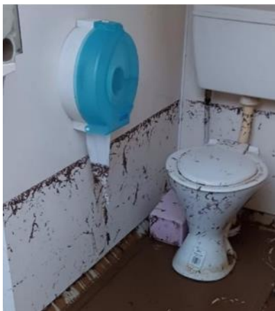
Figure 6: Toilet unit at Owen River Campground, showing the water line on the wall following recent flooding.
