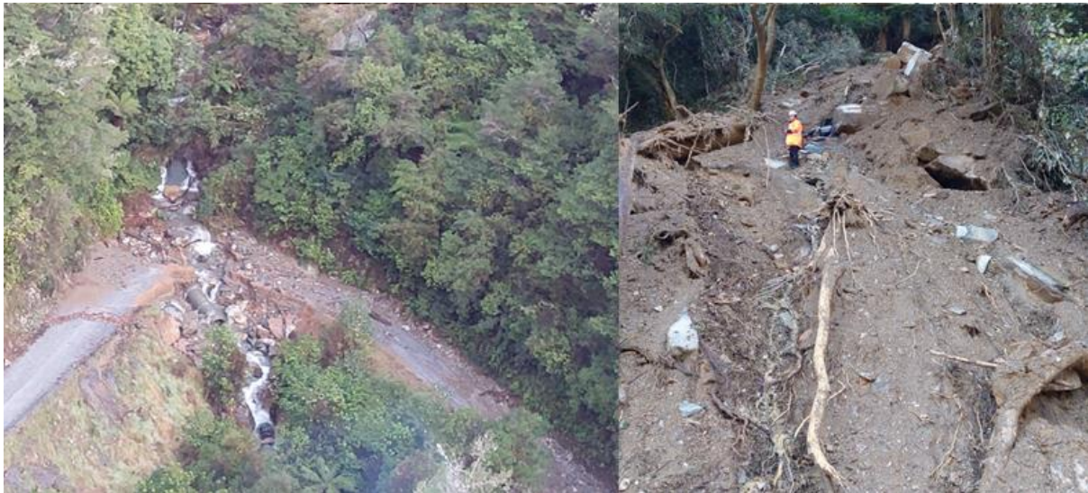
Figure 16 & 17: Cobb Dam Road, Culvert washout & major slip above the powerhouse
