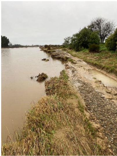
Figures 10 and 11: Erosion at Māriri closed landfill (L) and new rock erosion protection (R)
