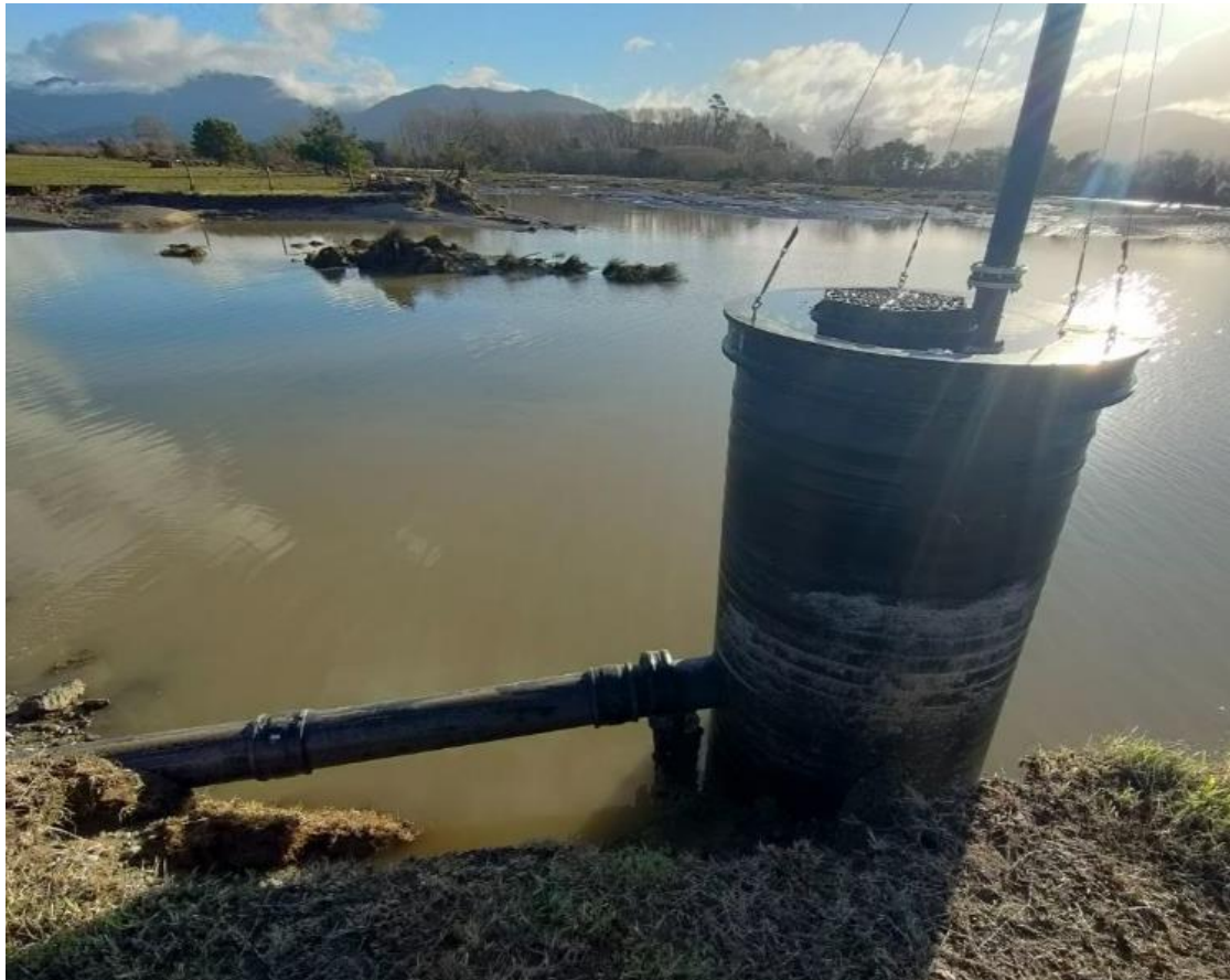
Figure 7: Damage to Motueka WWTP outlet structure
