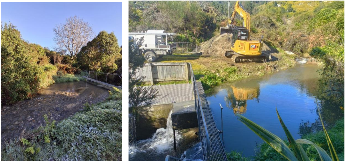
Figure 4: Winter Creek intake before sediment removal and after.
