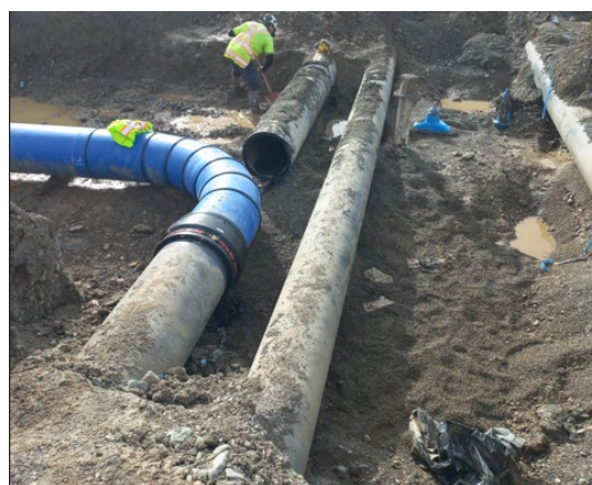
Cutover to the existing pipes
