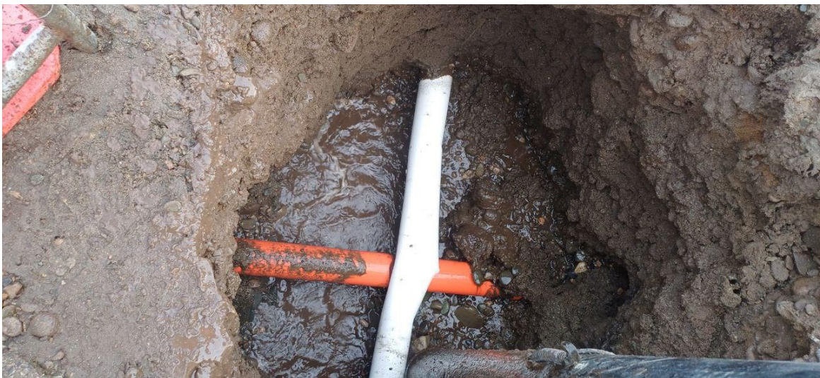
Figure 5: Service strike at Totara Park Avenue power duct install site
