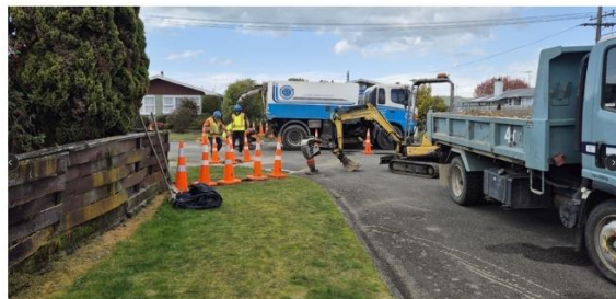
Potholing underground services on Woodlands Ave – a method of safely locating buried utilities before work begins.
