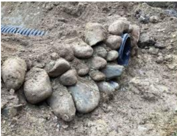
Matiri Valley Road – culvert 97 replaced
