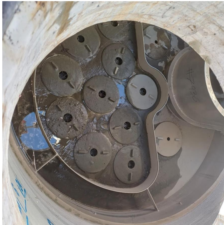
Picture 1: Jelly Fish Filter membranes viewed from the top
