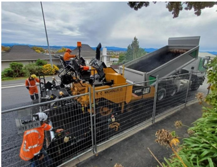
Picture 7 & 8: Rebuilding and asphalt application
