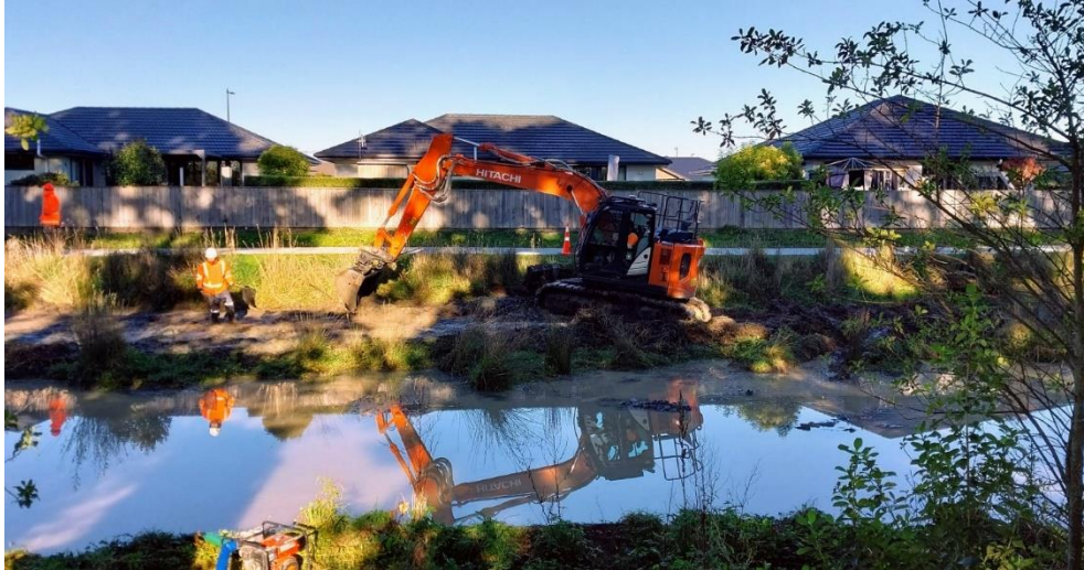
Figure 4: Poutama Creek physical re-shaping work
