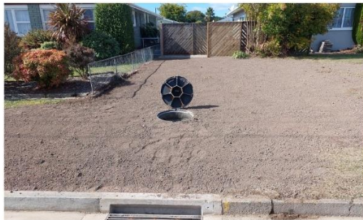
New manhole and stormwater sump – structures that provide access to underground pipes and collect rainwater runoff.
