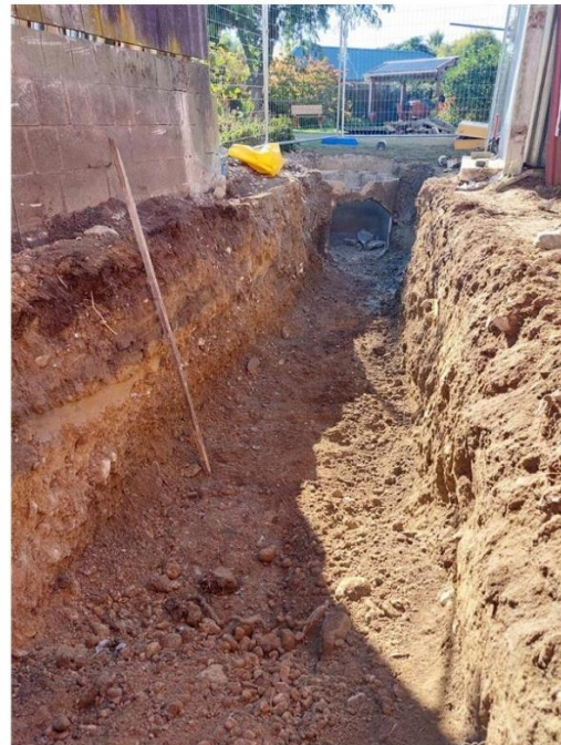
Before first pipe laid, this is a connection to the downstream manhole
