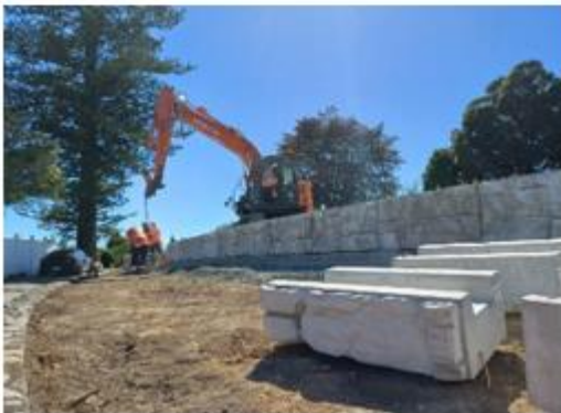
Picture Collection 9: featuring the magnum stone retaining wall.
