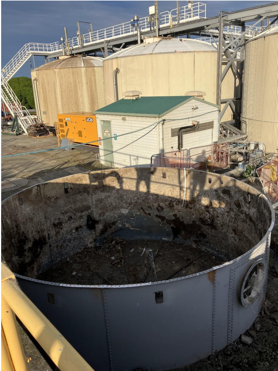
Figure 2: Old sludge storage tank with top strake removed
