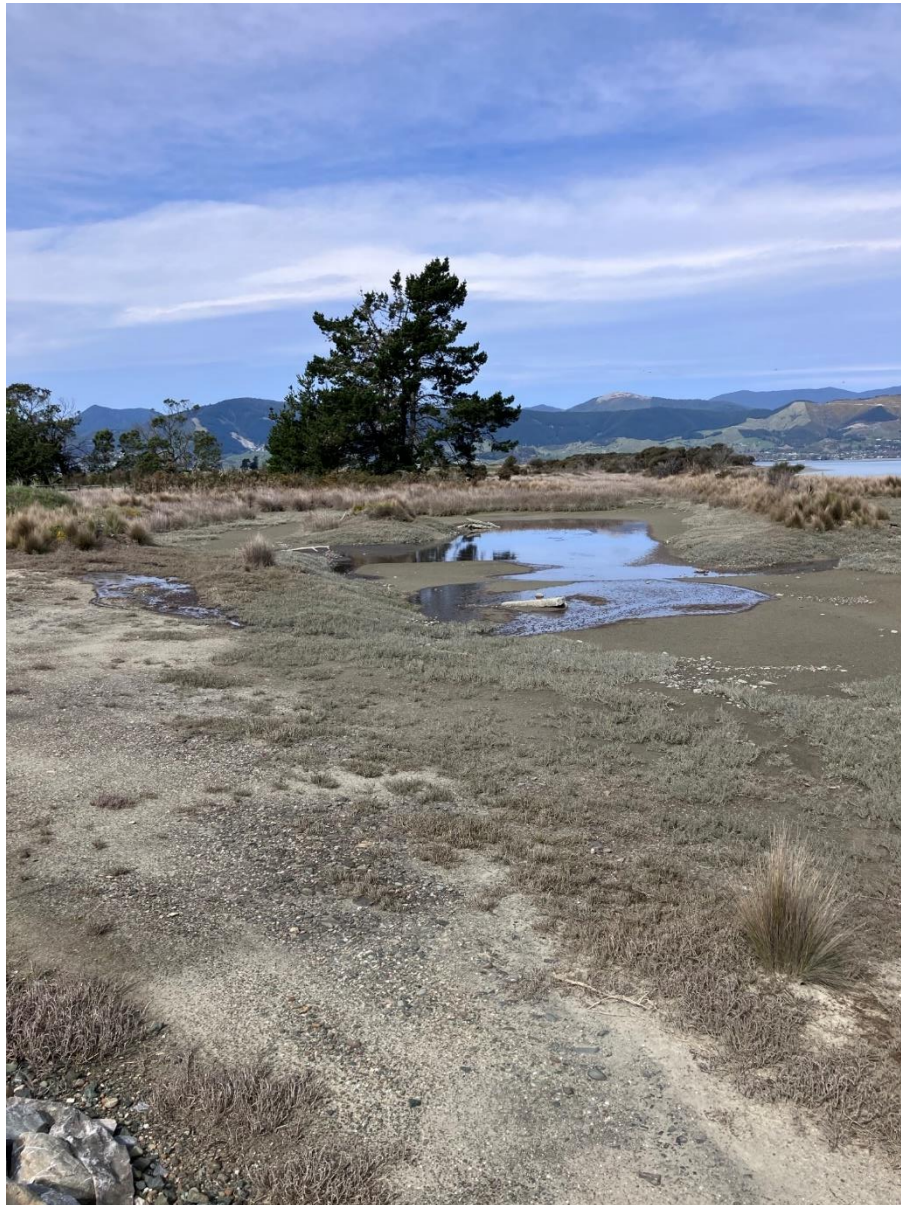
Figure 3: Biosolids pipeline failure site
