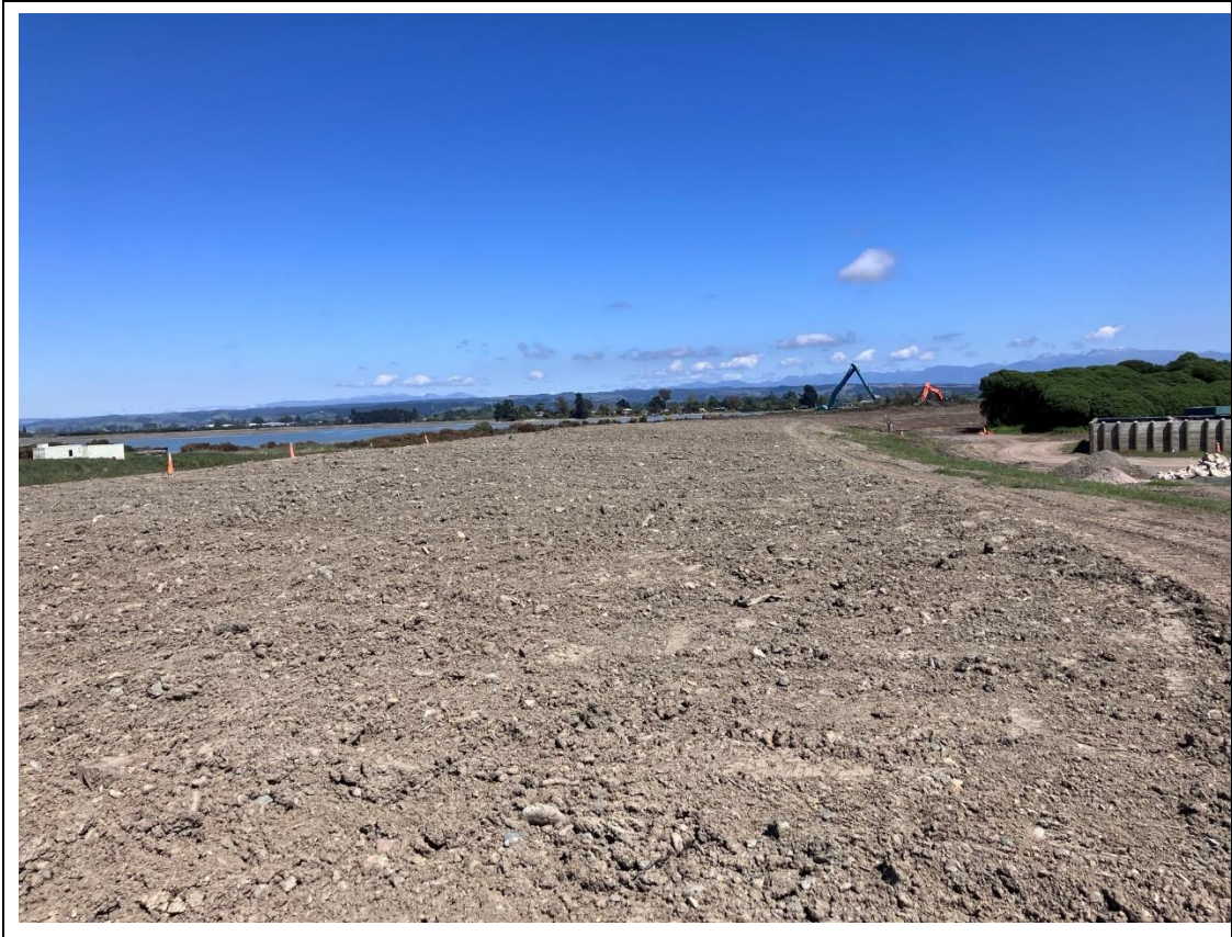
Figure 4: Covered sludge bund
