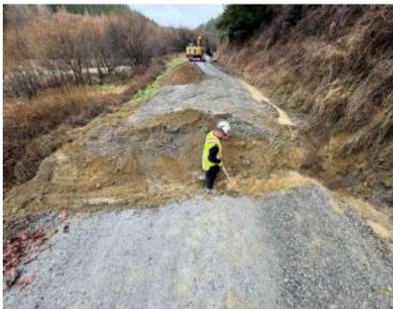
Howard Valley Road – culvert replacement
