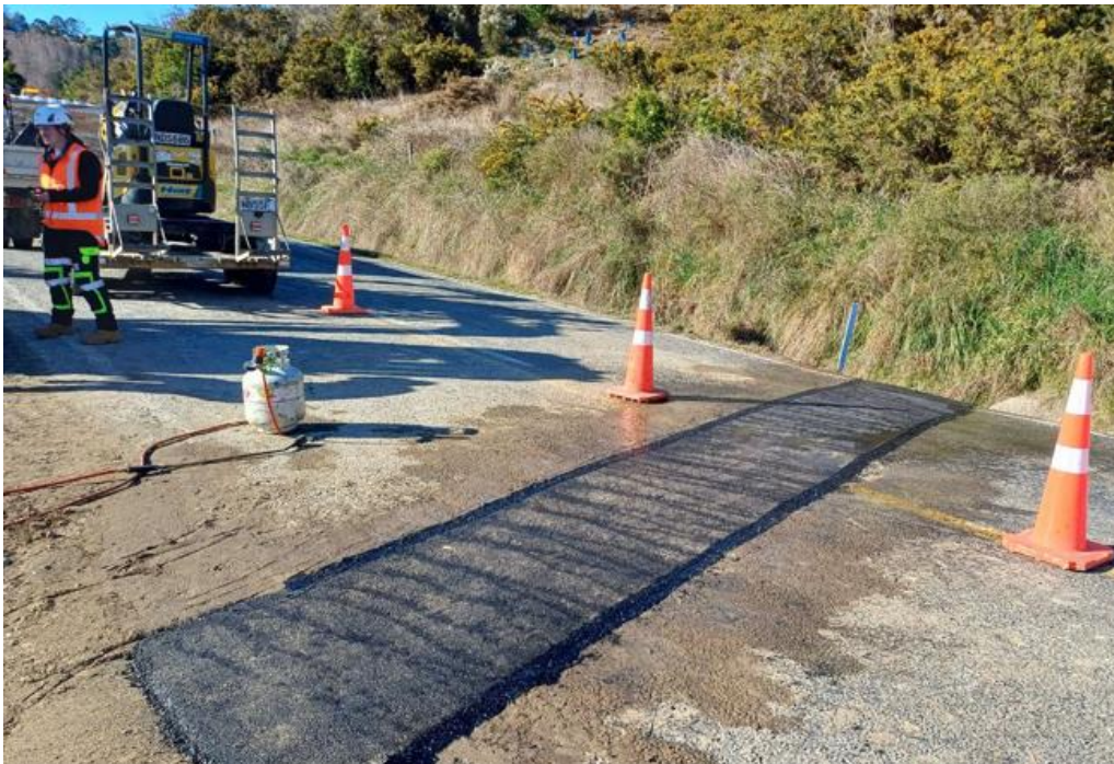
Picture 21 - Motueka Valley Highway culvert replacement
