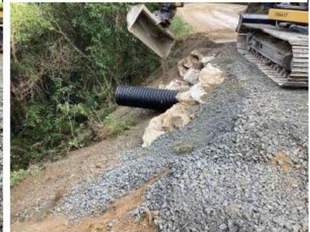
Aorere Valley Road – culvert replacement
