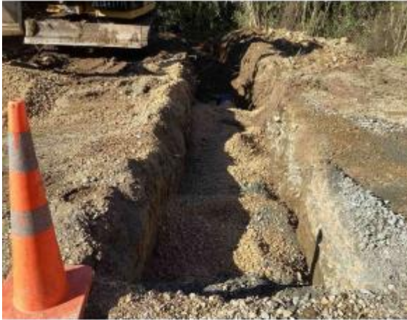
Aorere Valley Road – culvert replacement
