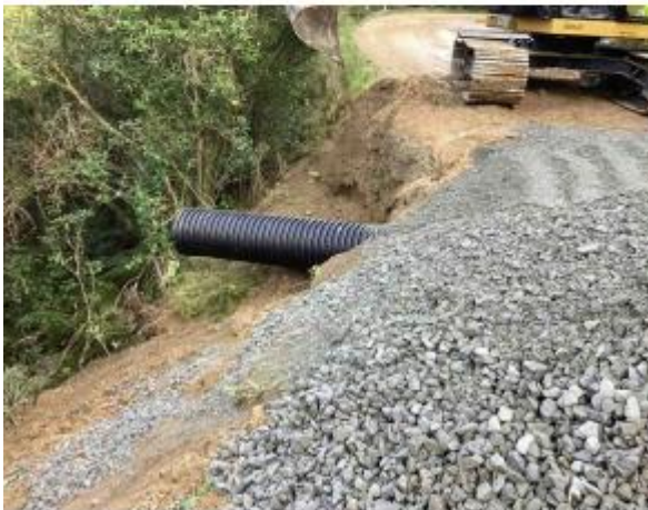
Aorere Valley Road – culvert replacement
