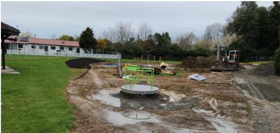
Picture 2: Progress of Faulkners Bush playground upgrade.
