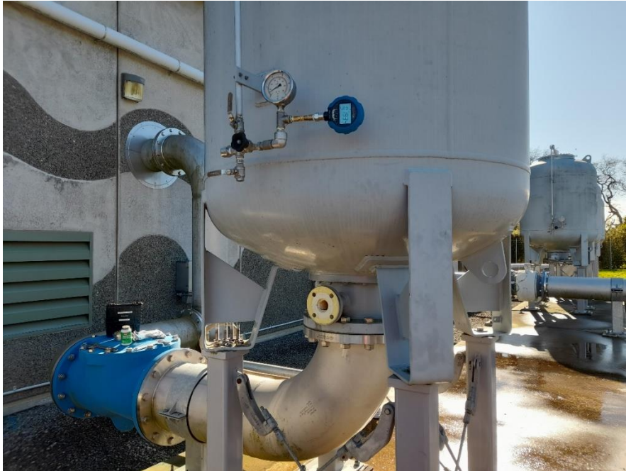
Figure 1: Richmond Water Treatment Plant surge vessel during maintenance
