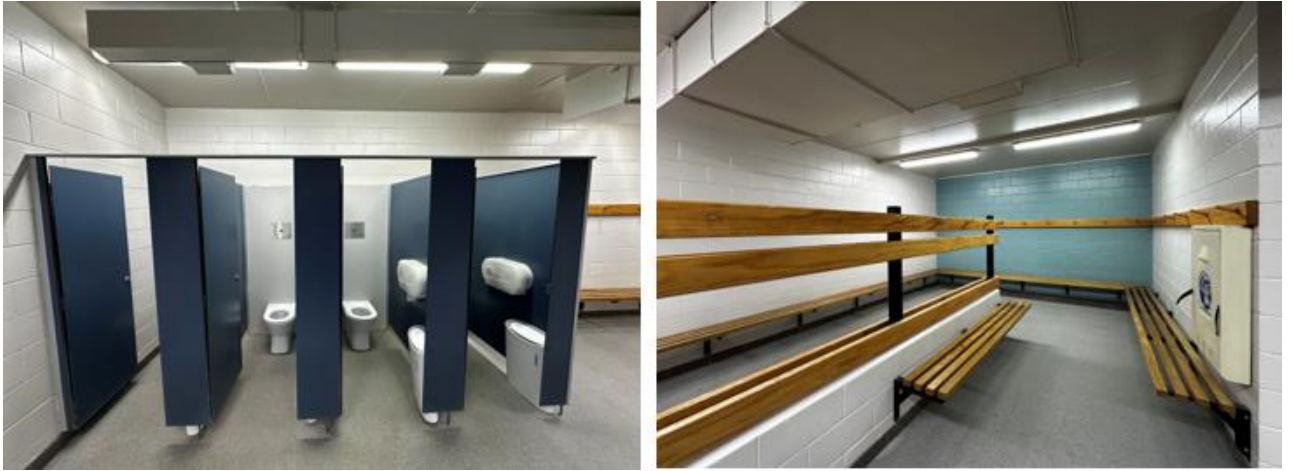
Picture 1 and 2: Recently completed toilets and changing room
