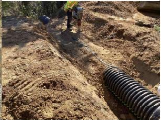
Aorere Valley Road – culvert replacement
