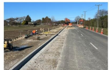
Pah St and Queen Victoria St Motueka (Underway)
