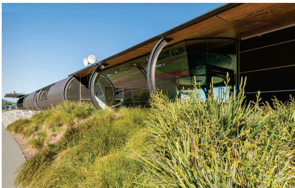
Figure 7 Saxton Oval Pavilion
