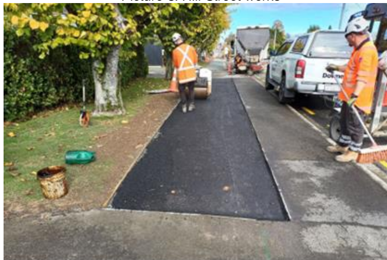
Picture 4: Rolling asphalt
