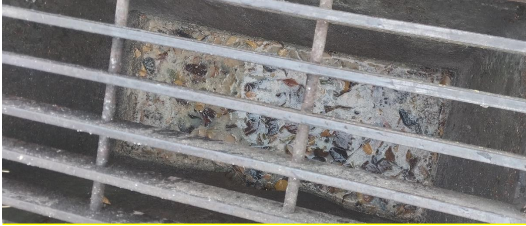
Figure 3: Looking down the contaminated sump showing a layer of grease amongst leaf debris.
