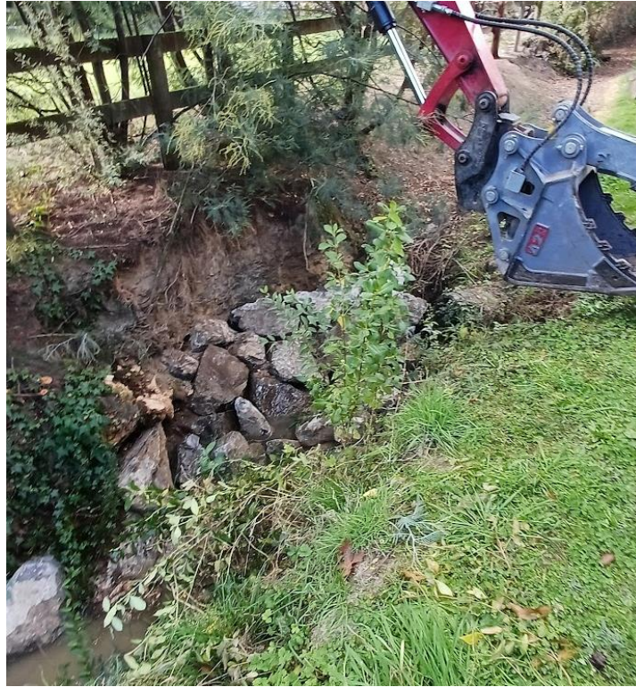
Figure 6: repairing bank scour on tributary of Reservoir Creek
