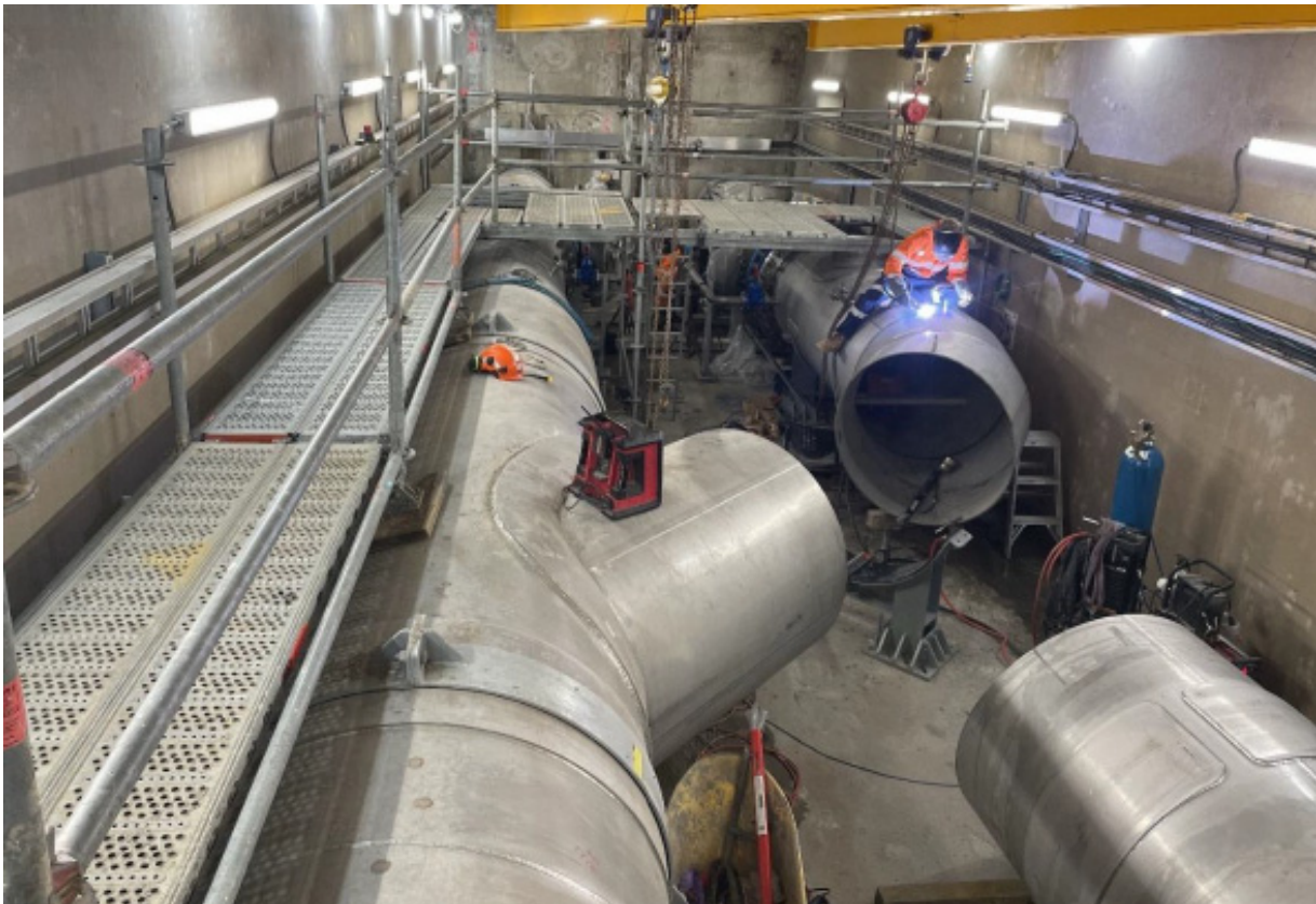
Figure 4: Welding pipework in the upstream culvert, February 2024.
