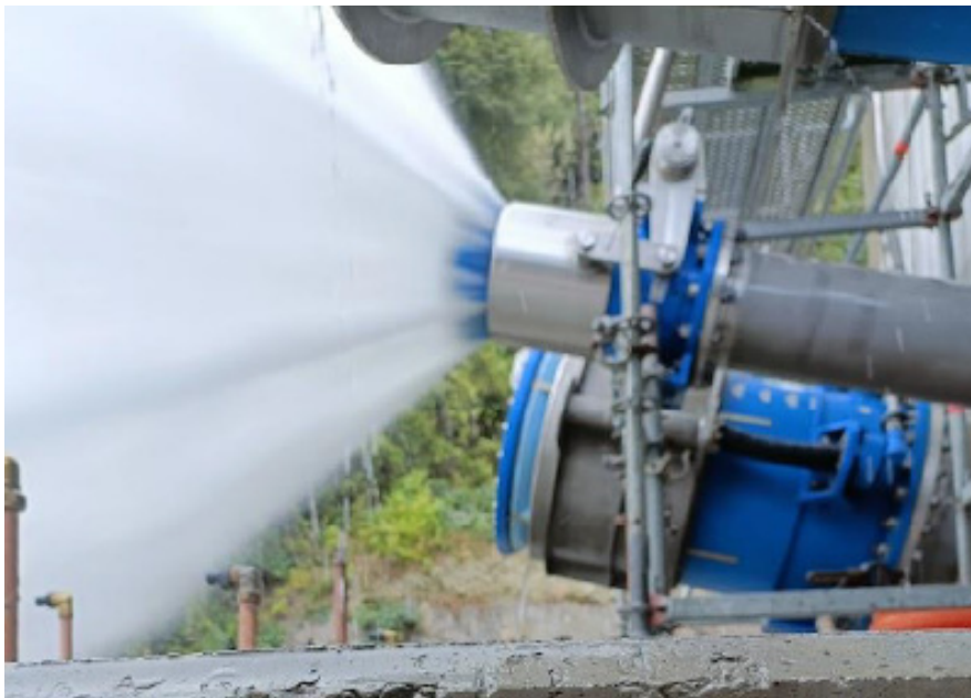
Figures 7 and 8: The small dispersing valve releasing water, 2 March 2024.
