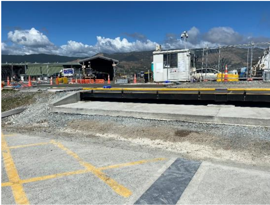
Picture 6: Richmond RRC weighbridge showing concrete base
