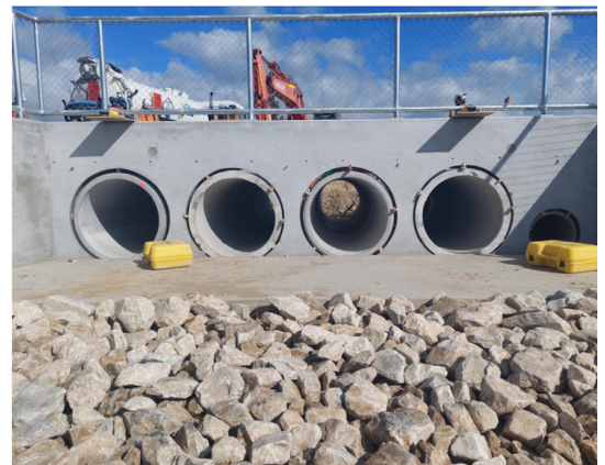
Outlet wingwall installed in Woodlands Creek
