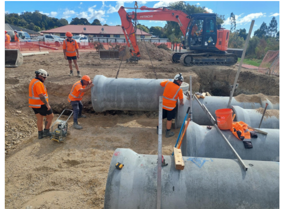
Workers installing culvert pipes
