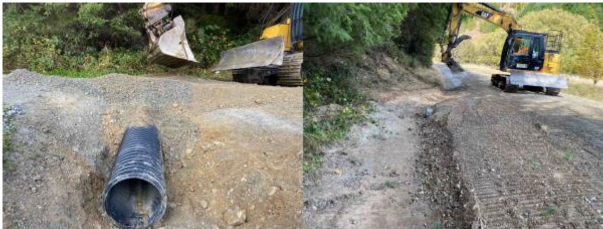
Higgins Road – culvert installation
