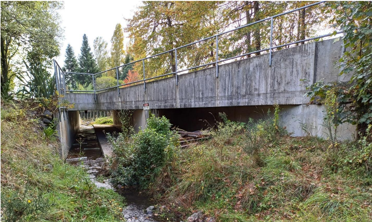
Picture 5: Champion Road culvert, with throttle plates removed
