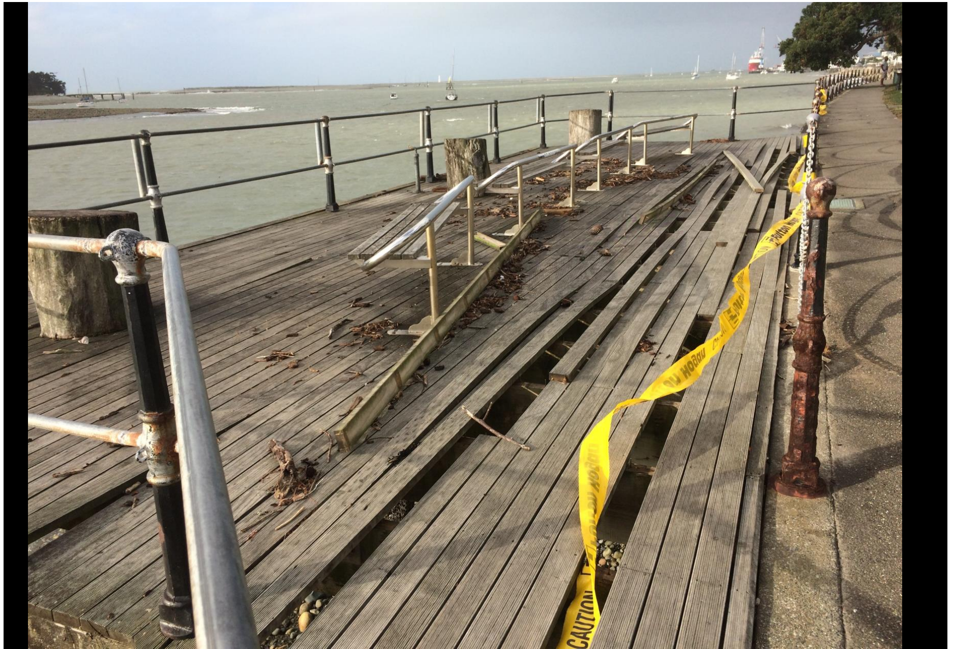
Topside of Fishing Platform after the cyclones
