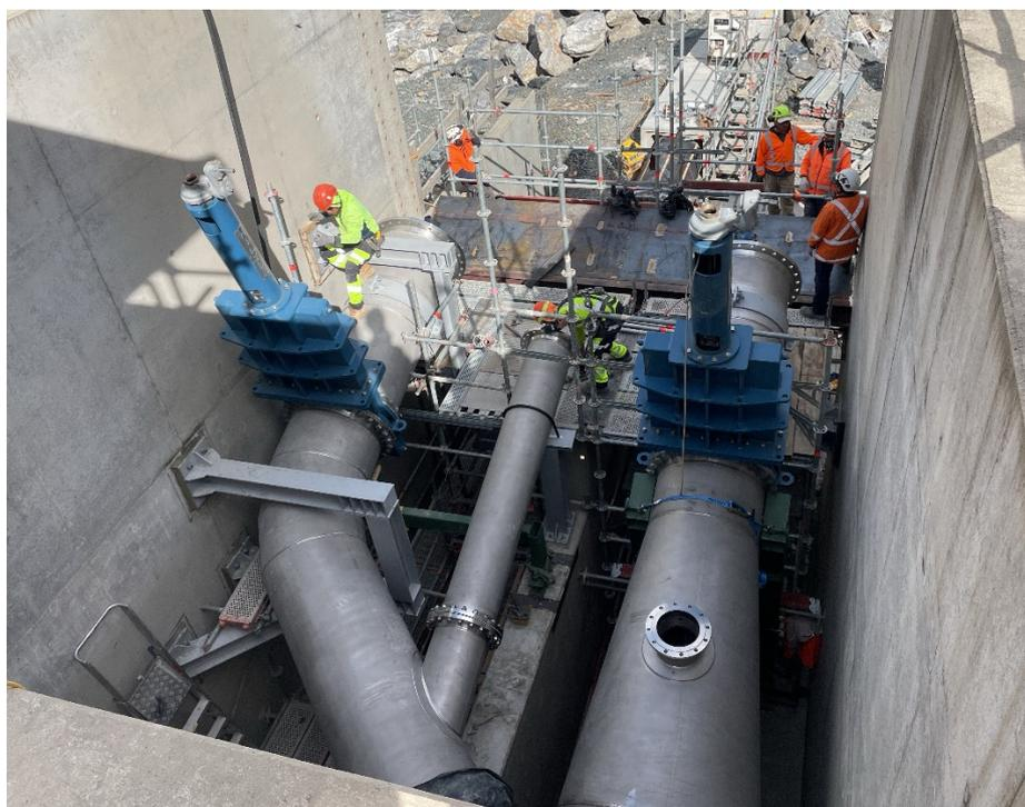
Figure 8: Permanent pipework in the right-hand side culvert being installed, December 2023
