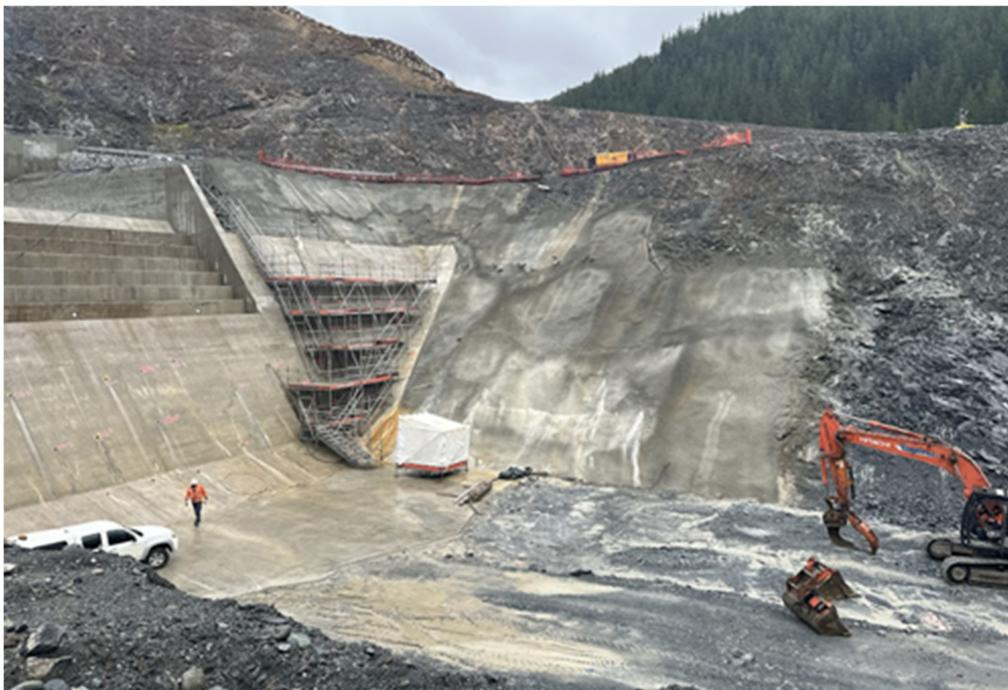
Figure 9: Plunge pool works being completed, October 2023
